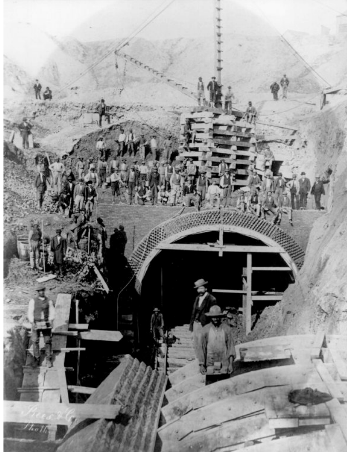
Figure 3. Construction of the Church Hill railroad tunnel, 1872. This massive excavation project cut through the Richmond deposit of diatomaceous earth, and provided C.L. Peticolas with substantial mounting material.
