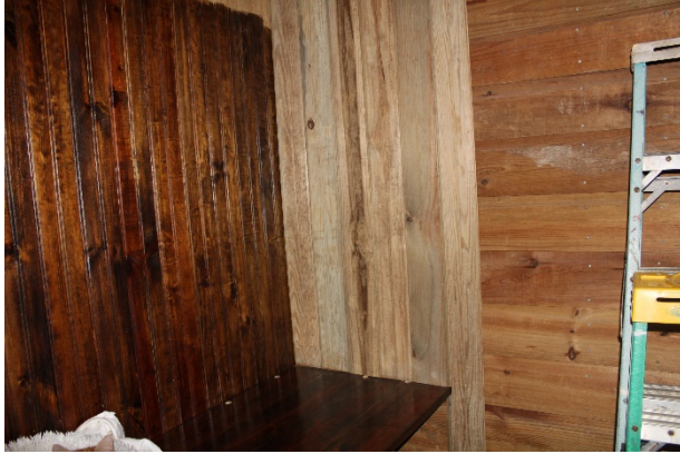
Unfinished bead board in place.
