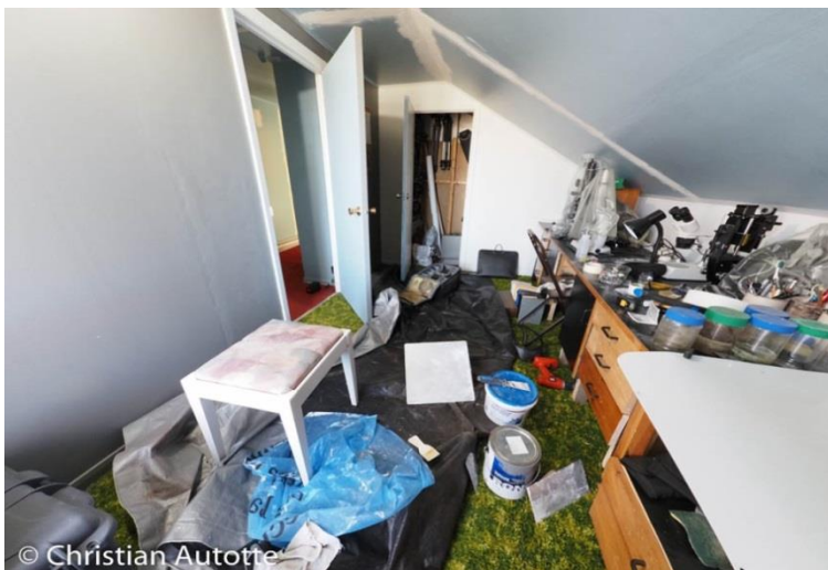
The studio during renovations, and once completed.
